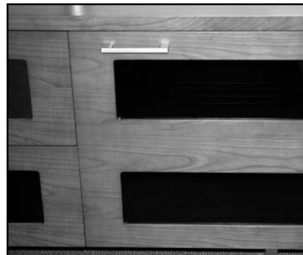
CORRECT! Door is sitting squarely and evenly spaced on tops and sides.
