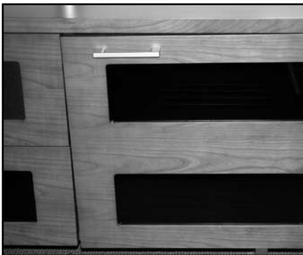
INCORRECT! Door is out of alignment with the rest of the unit.
