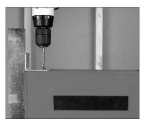
1. Attach brackets to the enclosure top and bottom on the side of the enclosure that will sit flush against the stud.
