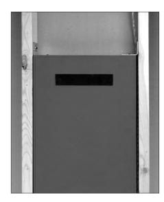
Place brackets top and bottom on the opposite side of the enclosure, then secure the brackets to the enclosure and stud.
