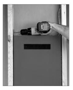
3. Place CSW155 in wall flush with stud faces, and attach tightened brackets to stud.
